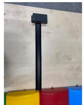
5. Now connect the speaker wire to the unit. Use the supplied cable + speakers + 2nd cable duct. The second cable duct does not need to be shorted. Install the cable duct on the wall again, exactly so that it falls over the terminal blocks. Install the speaker exactly above the cable duct.
