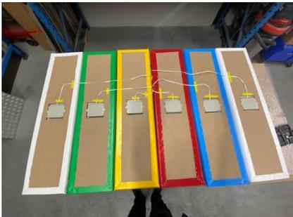
2. Install the panels on the wall using the mounting brackets supplied. Make sure that the wires come out in the middle at the top.
