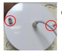
8. Align the metal cap with the protruding screws on the fixed metal bracket, then insert the nut and the screw cap to secure the bracket in place along with the metal cap.
